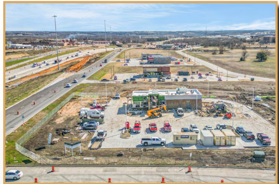
Construction Status as of January 2024
